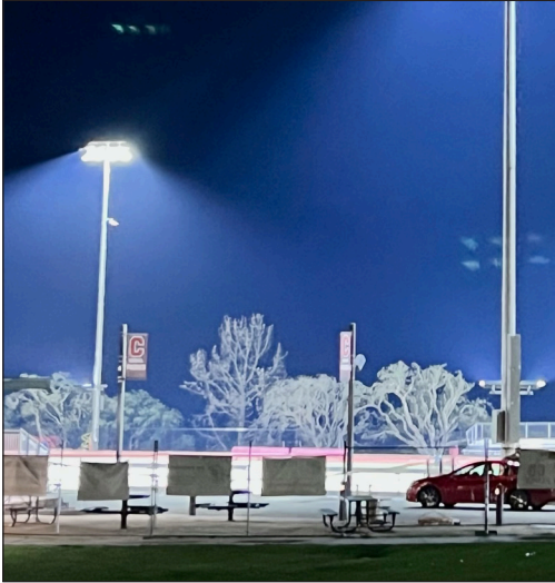
1) Downward-focused light beams from CHS's new stadium lights during Nov. 2023 tests –Photo: F. Dillard
